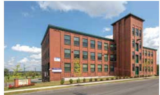
Harbor Street Lofts, a 40-unit mixed income historic project in Tipperary Hill.
